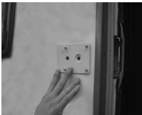
Mount inside backing plate and insert 4 screws
